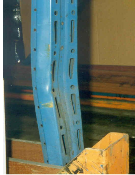
Fig. 17 Not allowed ("Red") damage. Immediate off-loading required
