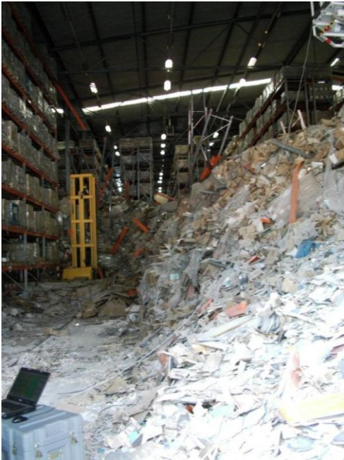
Fig 12. Example of a the result of a progressive collapse
